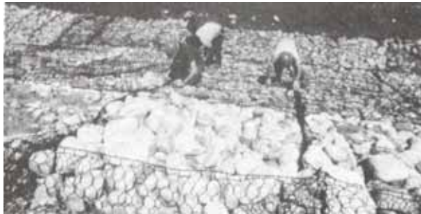
Exhibit XIII .6 Wire Enclosed Rock Riprap
